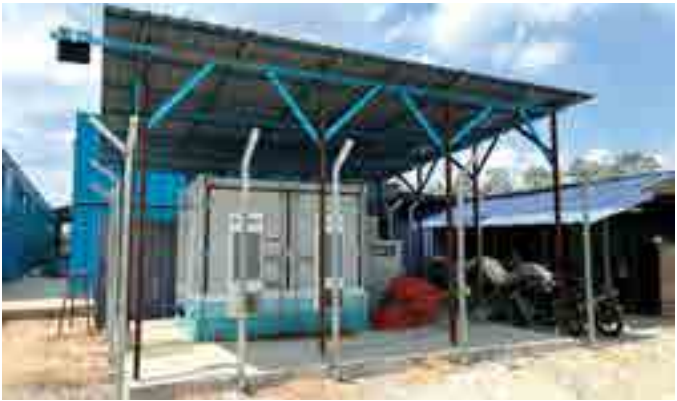
Battery Energy Storage System
