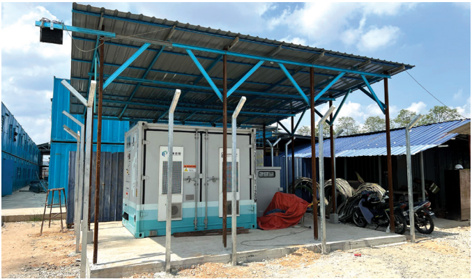
Battery Energy Storage System
