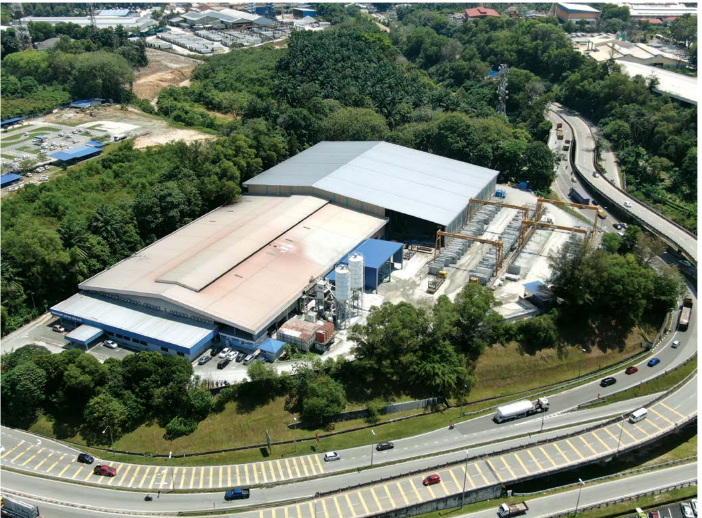
IBS Precast Concrete Factory, Nilai
