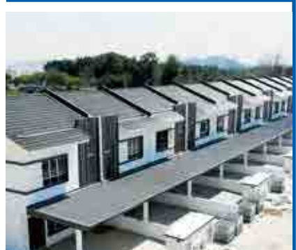
Pilot IBS Precast Concrete Project @ Alam Perdana
