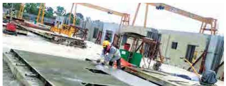
Precast Concrete works in Alam Perdana's mobile plant
