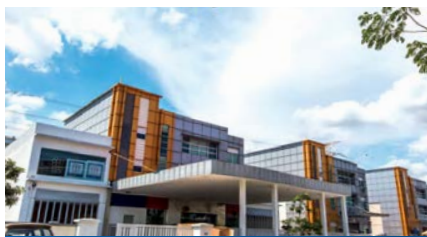
Taman Tasik Puchong Industrial Park -3 Storey Bungalow Factory
