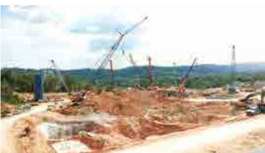
Piling work for Residensi Bintang @ Bukit Jalil
